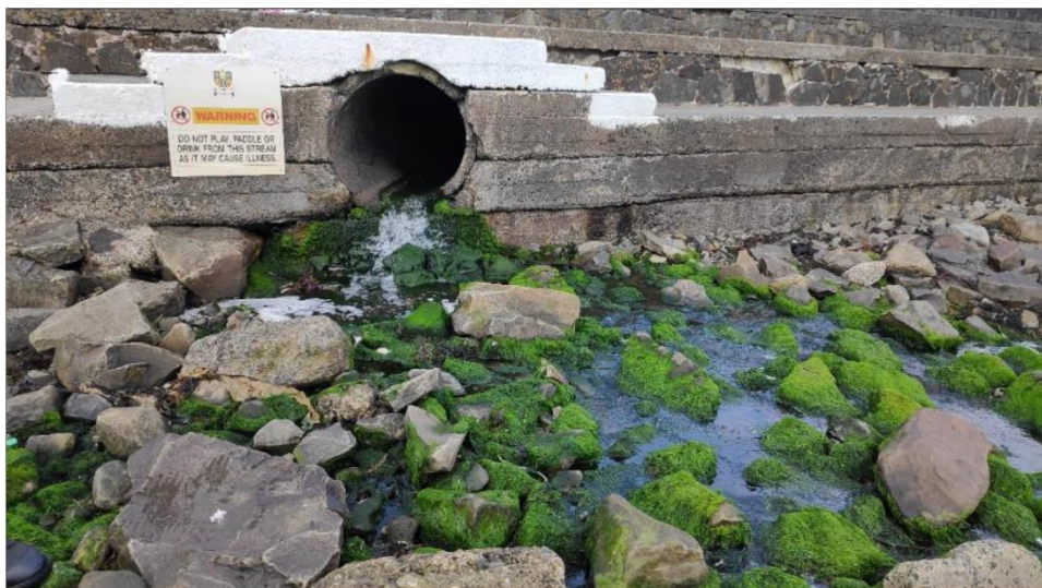
Plate 3.12 Outfall of the unnamed stream ('Atlantic Stream') to the sea near Kilkee Pier, 0.4km downstream of site 5 (significant fish passage barrier)
