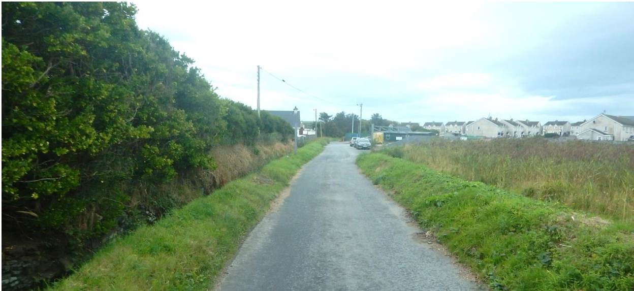
Figure 12-8: Existing Well Stream open channel on the left of the existing local road.
