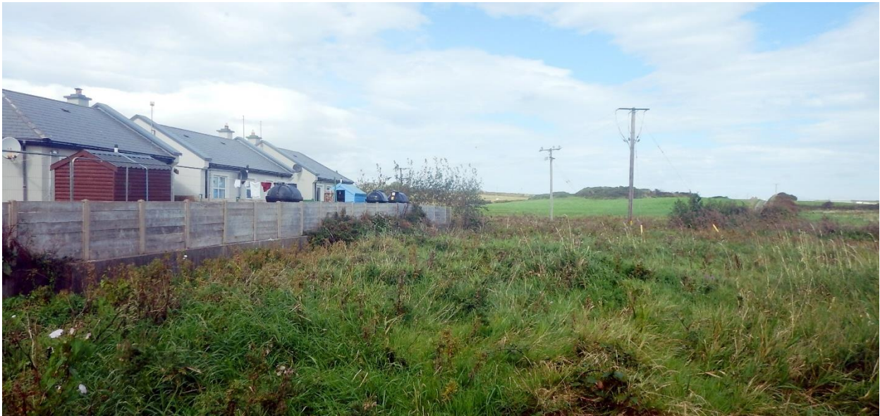
Figure 12-2: Existing rear boundary to residential dwellings adjacent to Atlantic Drain #2 and the Atlantic Stream.
