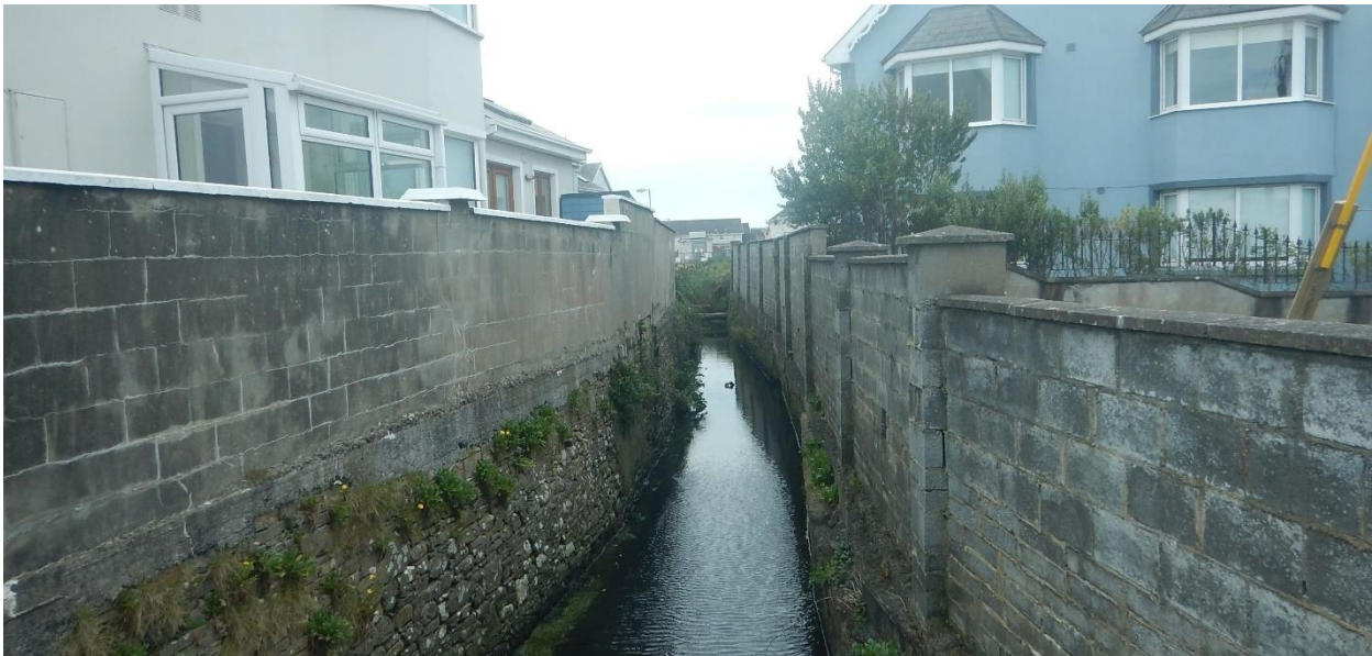
Figure 12-7: Existing the Victoria Stream open walled channel.
