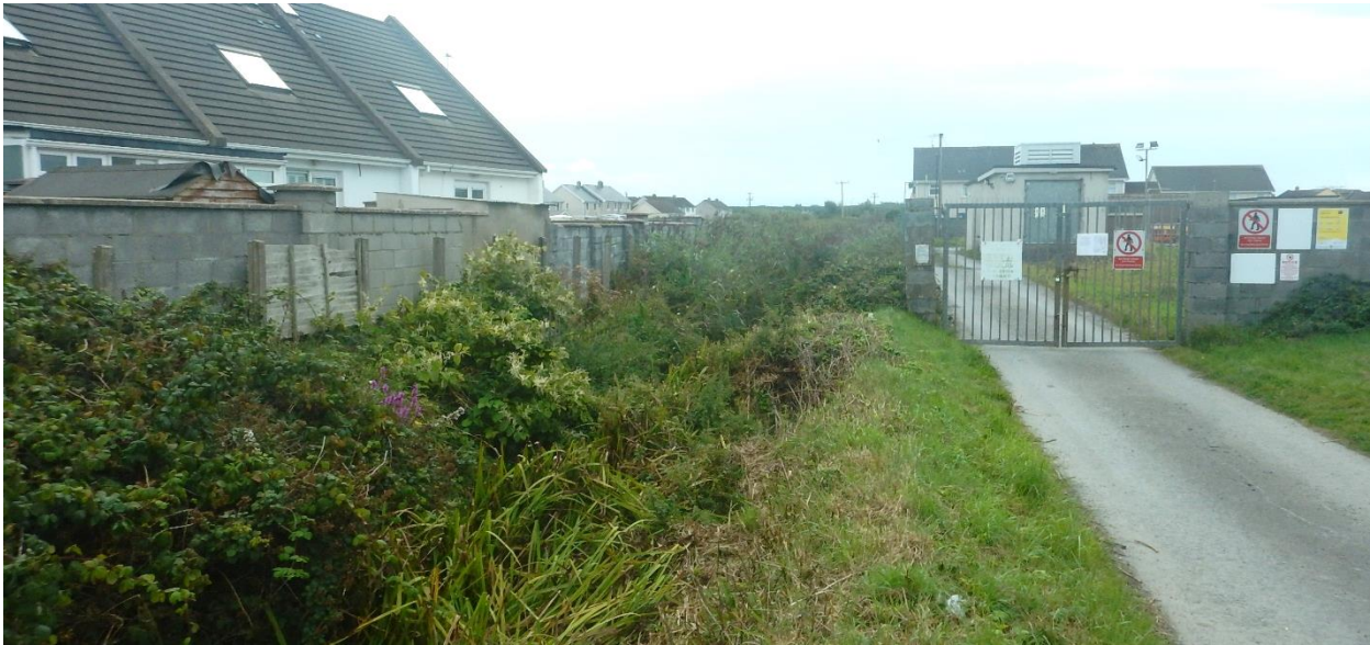
Figure 12-6: Existing the Victoria Stream ditch and overgrown vegetation.
