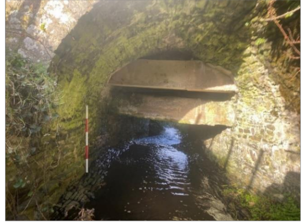
Interior of stone arch with crossing services taken from the southeast.
