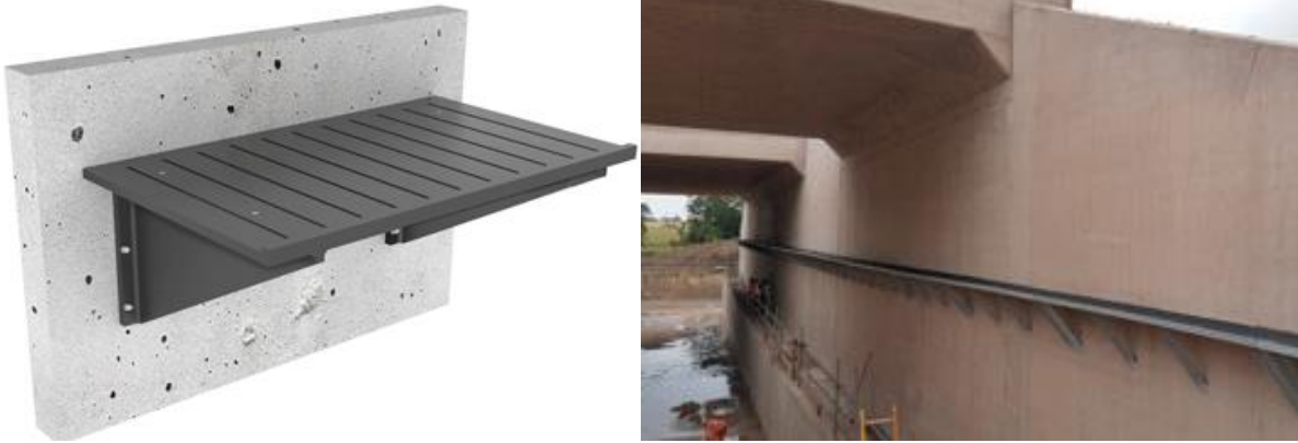
Figures 7-37: Example of mammal ledge (left) and aspect of installed ledge (right) 134 .
