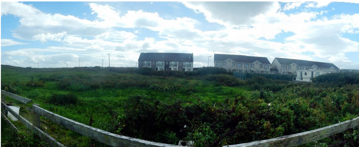
Figure 12-3: Existing southern boundary of Kilkee Bay Hotel, adjacent to Atlantic Drain #2.
