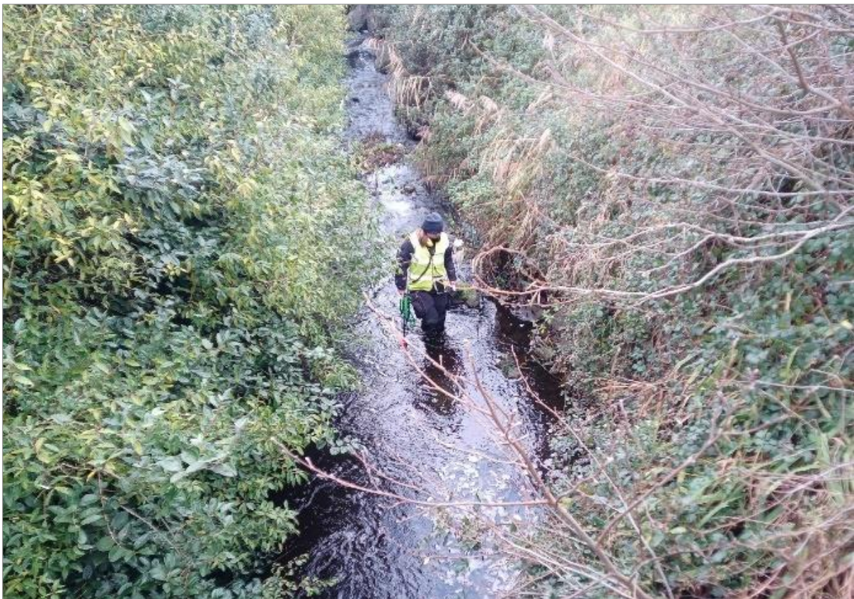
Figure 11-1: Working shot of wade and metal detection survey of Atlantic Stream from the SE.
