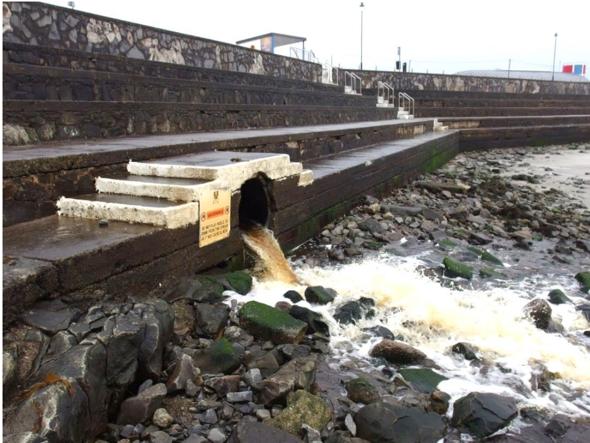
Figure 7-10: Atlantic Stream culvert main outfall
