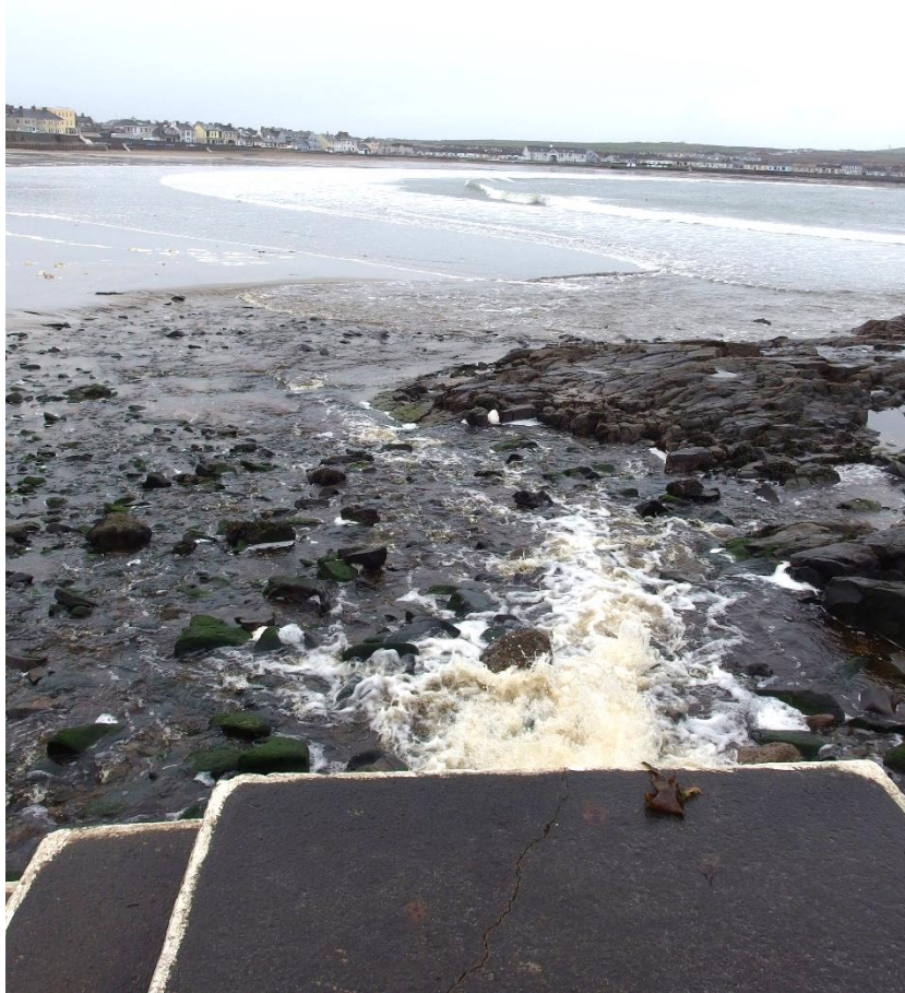
Figure 5-8: The path of the water from the Atlantic outfall is skirting around the more intact reef areas.
