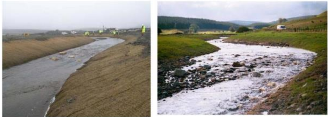
Figure 8-4: Use of biodegradable matting can protect sediment release from soil erosion, but allow natural regeneration of vegetation (from SEPA 2009).
