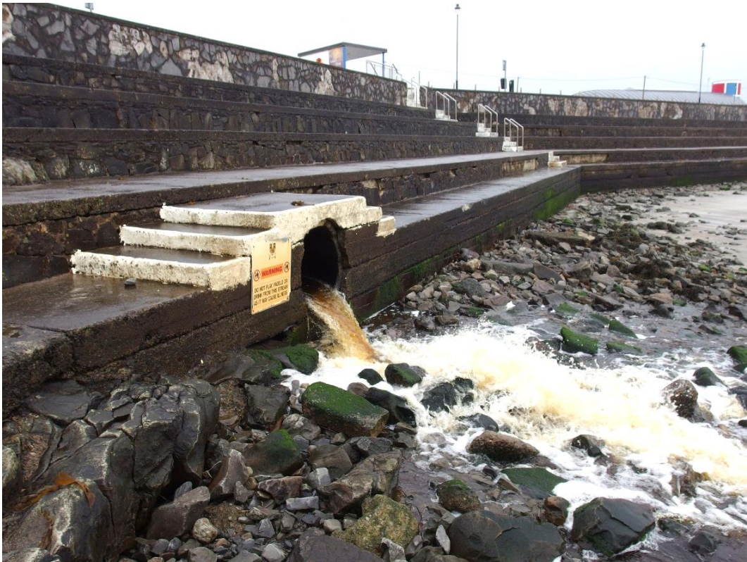
Figure 5-2: Atlantic Stream culvert main outfall.
