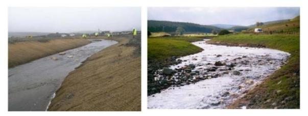
Figure 6.5: Use of biodegradable matting can protect sediment release from soil erosion, but allow natural regeneration of vegetation (from SEPA 2009)
